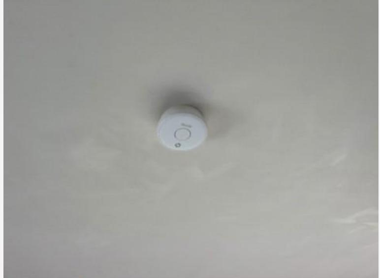
The hallway smoke detector was not working at the time of this inspection
