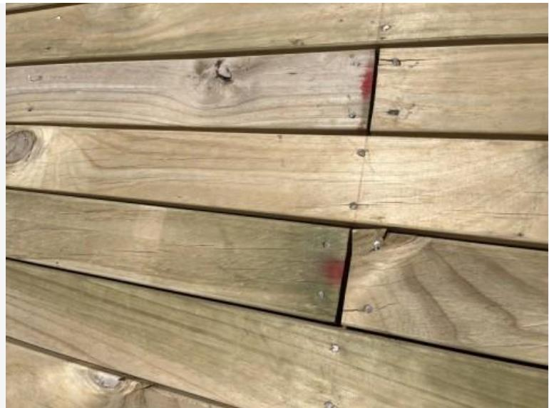
Squeaking was noted from the decking boards when walked on. A decking board also appeared to be in contact with a pipe adjacent to the deck. Uneven clearance was observed around the pipe penetration, with some sections too close to (or in contact with) the pipe. This may contribute to noise, ongoing movement, and potential wear to the decking and/or pipe over time.
