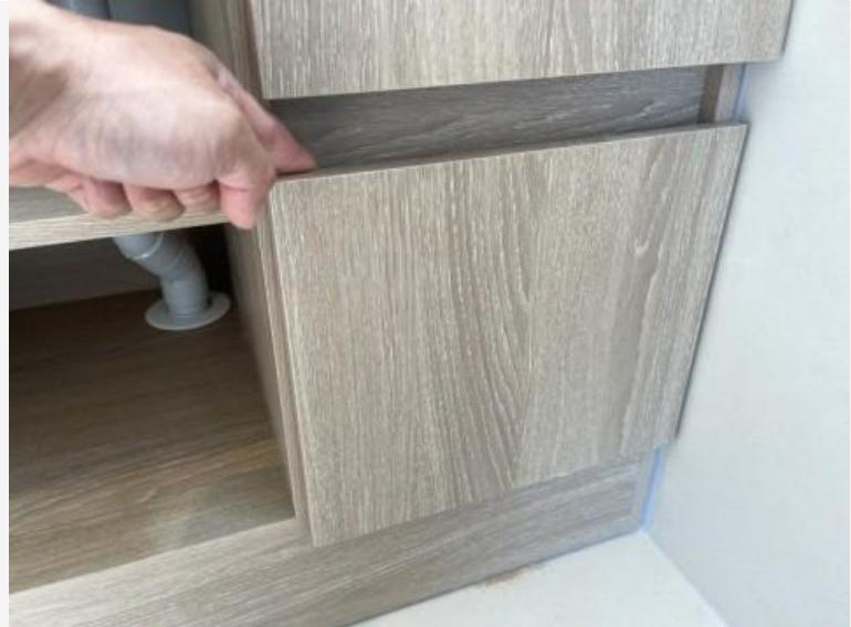
A drawer was observed to be off its runners and did not operate correctly at the time of inspection. Recommendation: Have the drawer runners assessed and repaired/adjusted by a cabinetmaker or competent tradesperson to restore safe and functional operation.
